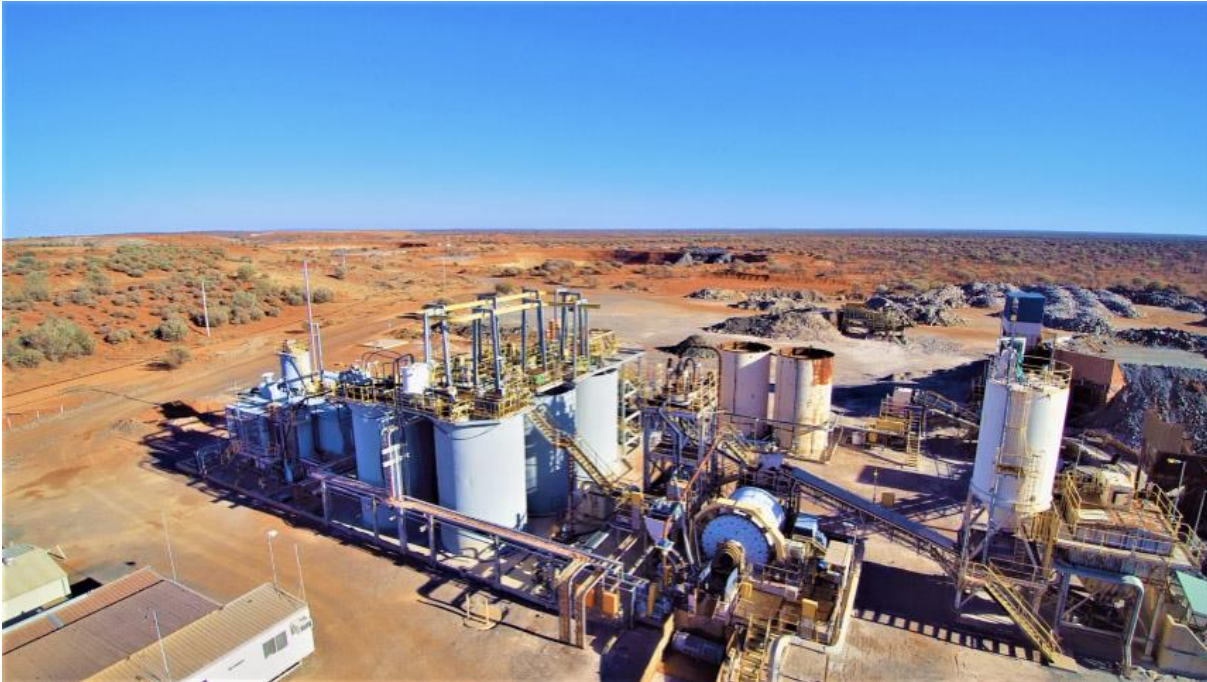
Figure 2 - Burnakura gold processing plant
